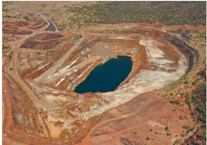
Looking south at the nearly dewatered Batman pit. Scale varies with perspective.
